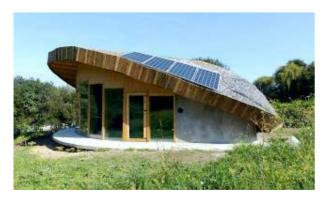
Biovalvo module built with recycled mussel shell
